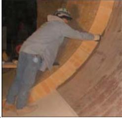
**Background:** Producers of lime and Portland cement operate rotary kilns as part of their manufacturing process. These rotary kilns are large horizontal cylinders, slightly elevated at the charge end to permit gravity to propel their product through kiln, which rotates slowly to tumble the product inside the kiln. Operating continuously at very high temperatures, these rotary kilns are lined with dense refractory blocks to protect the steel casing (shell) of the kiln from the high heat.
